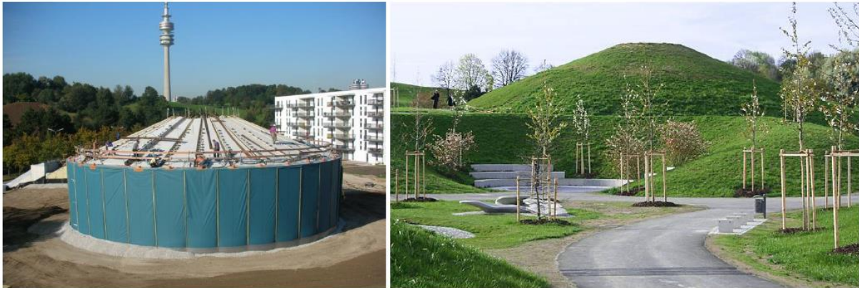
Figure 30 - TES with 5,700 m 3 of water volume built from prefabricated concrete elements in Munich, Germany (in construction and finalized, Solites).
