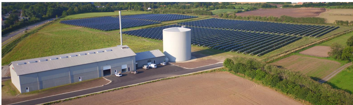
Figure 29 – TTES of 3,000 \text{m}^3 in Hjallerup, Denmark in connection to a solarfield of 21,500 \text{m}^2 and a straw boiler of 1.8 MWt (Hjallerup Fjernvarme).
